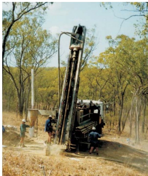
Nymbool Gold Project - DRL Drilling
